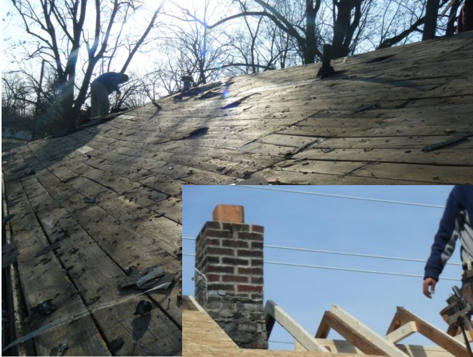
Above: Tearing off an old roof.
