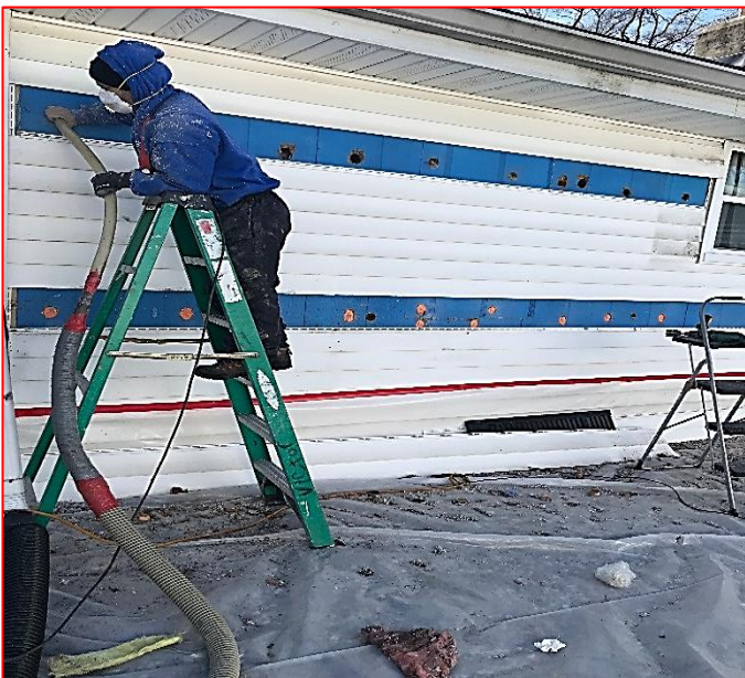
CAGI's Weatherization Program Contractor installing insulation. (left and above).
